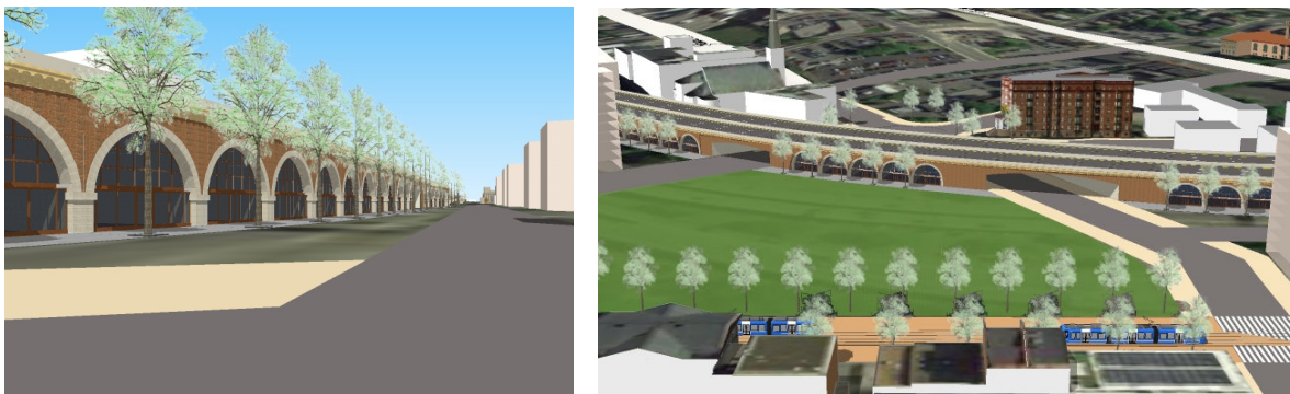
Figure 4: Example I-690 archway viaduct (1) looking east along re-established Canal St from corner of State St; and (2) looking north across the new Canalway Park (State St and “Erie Way”), an area previously under the spaghetti junction. Each archway would be 30-35ft wide.
